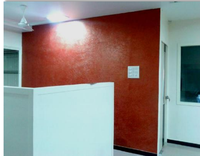
Wall Paneling - (V-Board)
