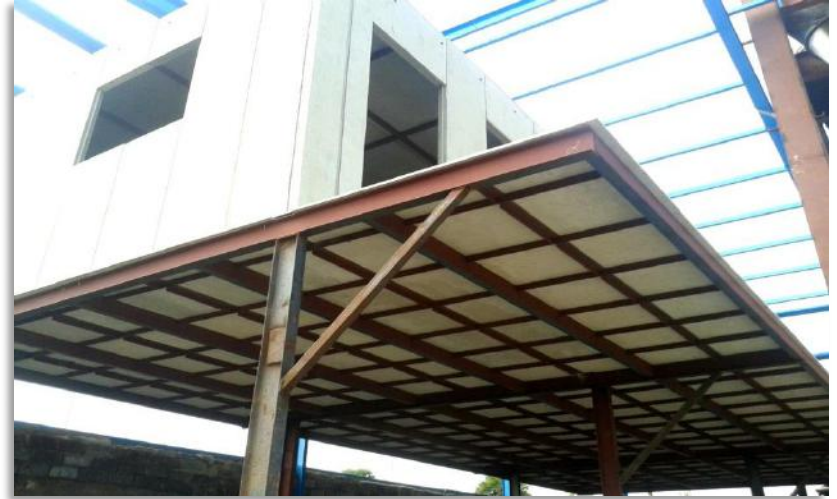
Mezzanine flooring - (V-Board)
