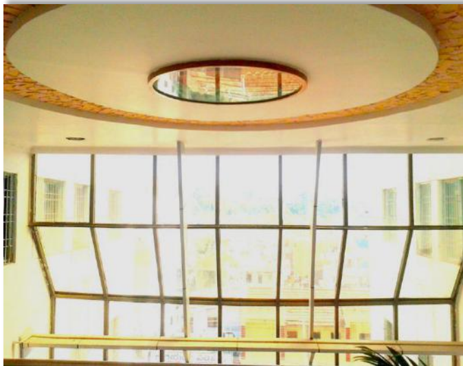
Concealed Grid False Ceiling - (V-Board/V-Designer)
