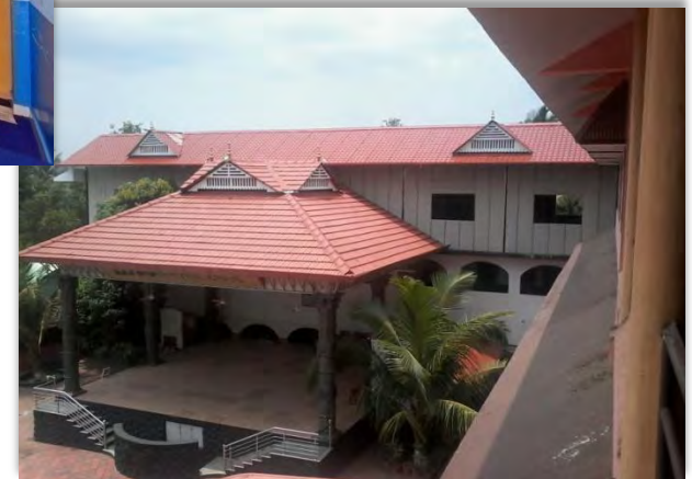
Roof Top Extension - (V-Panel )
