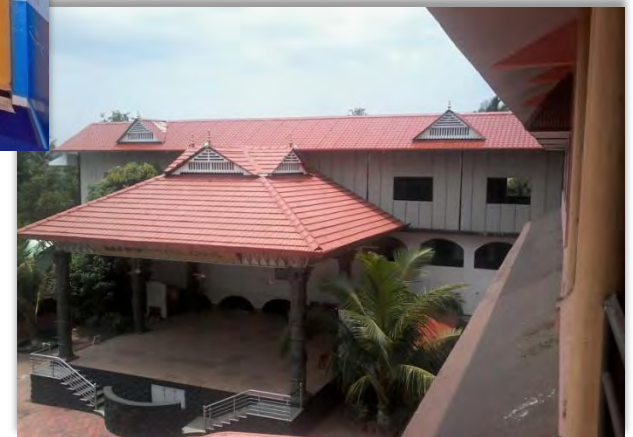
Roof Top Extension - (V-Panel )
